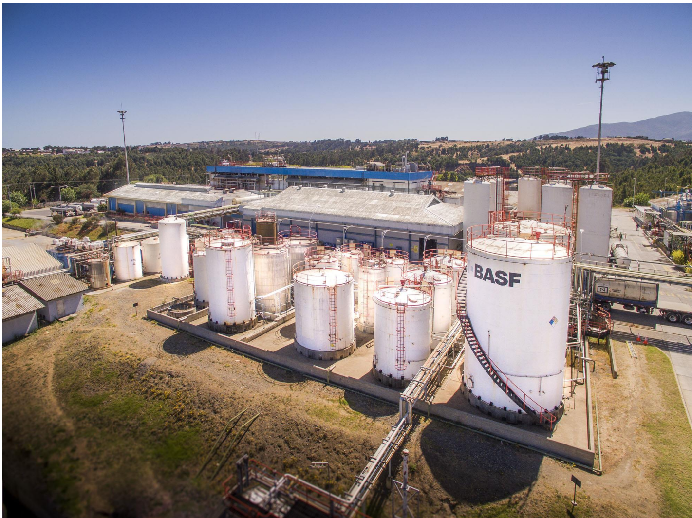
Concon Plant, Chile.
